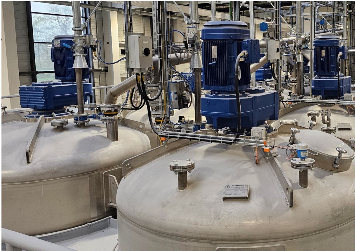
Storage of finished products in large tanks at KLB Kötztal.
